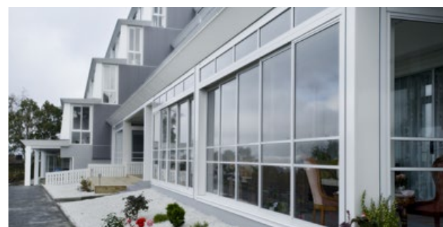
Balco's Etage solution is used for glazing stepped balconies
