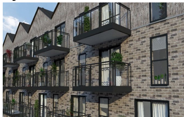
New Road Rainham, UK
